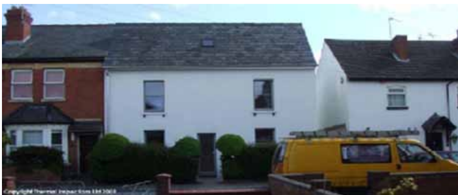
Simmonds.Mills / Thermal Inspections Ltd
