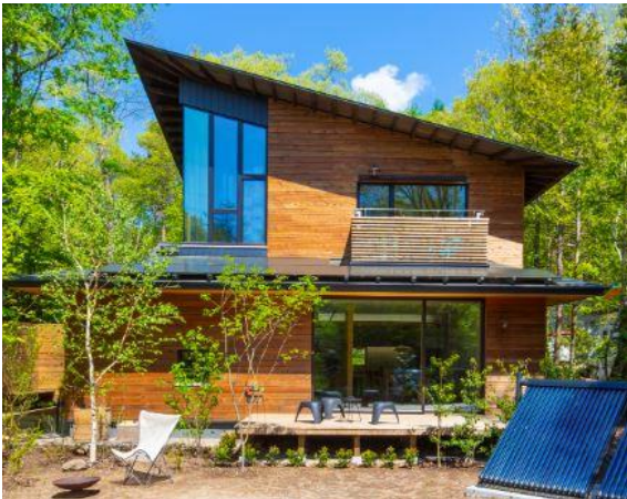
This Passive House building with solar thermal energy and PV system is open for viewing in Nagano, Japan. ID 7158 © Key Architects
