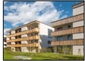
Apartment blocks to the Passive House standard. © Neue Heimat Tirol
