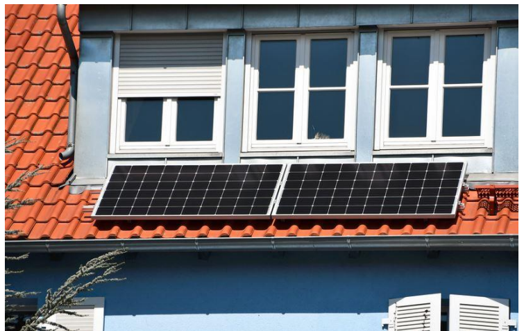
Small scale PV is one measure to save fossil fuel. In Germany, these so called "plug solar devices" only have to be registered with the grid operator. © Jörg Sutter
