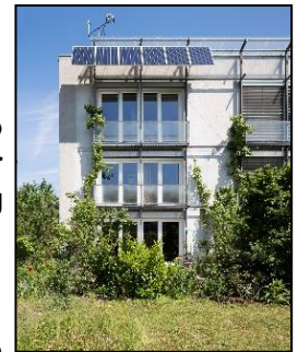
The world's first Passive House building in Darmstadt. © Peter Cook
