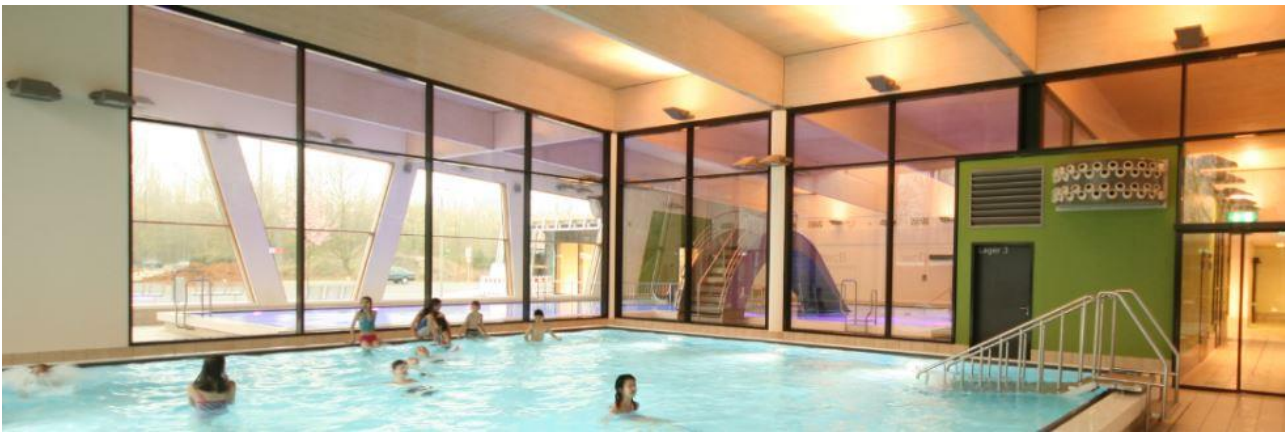
The Lippe-Bad in the town of Lünen in Westphalia is seen as a pioneering project for the Passive House Standard for indoor swimming pools. The handbook which has now been published is also helpful for already existing pools. © PHI
