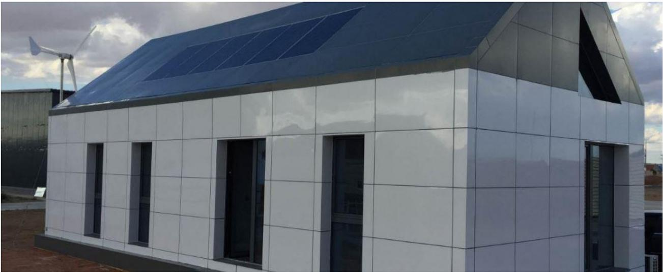
The shipping containers after conversion. The façade of the Passive House pilot project consists of anodised aluminium panels which reflect the countryside. In winter the floor slab can store heat for a long time and helps keep the building pleasantly cool in summer. In Mongolia the rural population will be provided with comfortable housing in order to reduce migration to cities. © Ludwig Rongen
