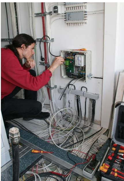
Passive House Institute staff installed numerous cables and sensors for the subsequent monitoring. Right: Ventilation pipes in the corridor of the administrative building in Baunatal. Photos: Passive House Institute
