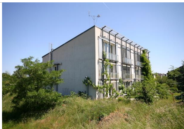
The world's first Passive House building in Darmstadt-Kranichstein.
