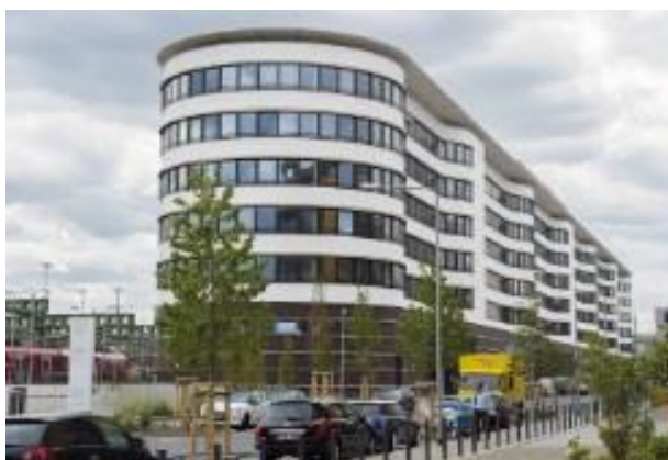
The new administrative building in Frankfurt, Germany, built to the Passive House Standard. Photo: City of Frankfurt
