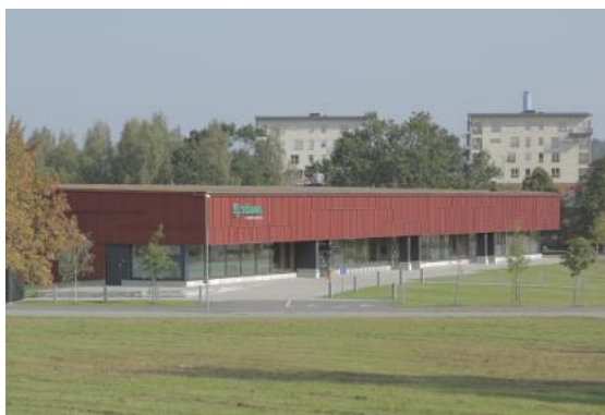
The "Södra Climate Arena" in Växjö – first of its kind in Passive House Standard. Photo: Günter Lang
