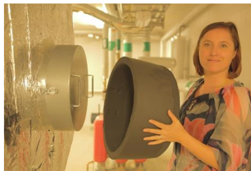
Energy consultant Simone Kreutzer checking the building services. Photo: Günter Lang
