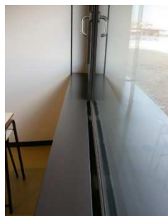
Ventilation slit for fresh air from outside at the windowsill.
