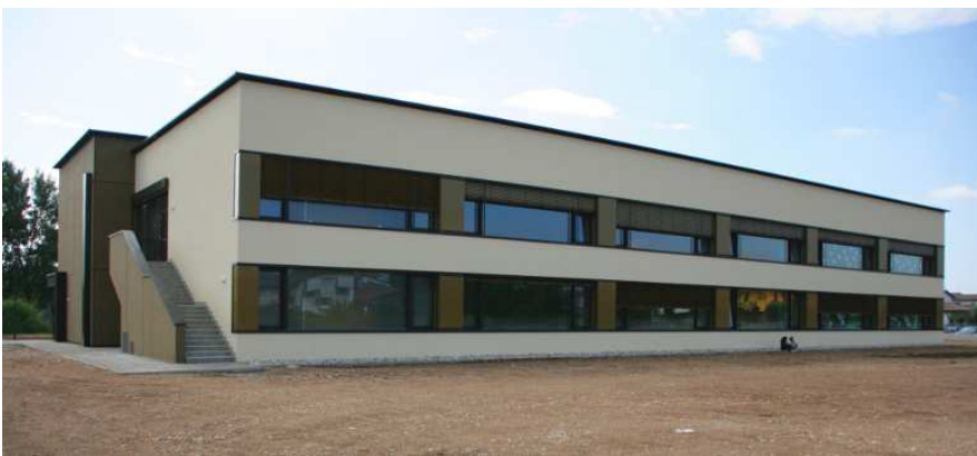
The primary school in Raldon opened its doors in September. The Passive House certificate is a guarantee of its superior efficiency. Photos: Passive House Institute
