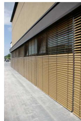
Detailed view showing shading elements.
