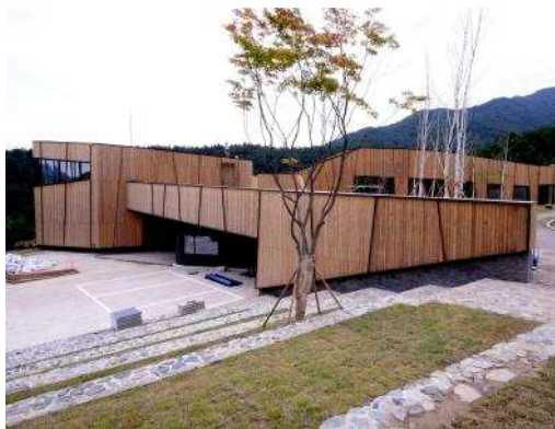
The educational centre is the largest Passive House in South Korea. Picture: Pulmuone
