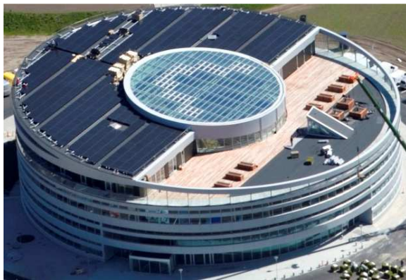
The new Passive House Headquarters in the Danish port city of Esbjerg. Photo: SE / Hoffmann A/S
