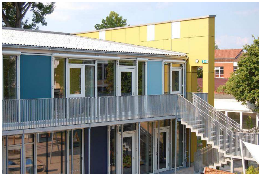
Passive House kindergarten in Hannover-Linden, Source proKlima/Glombik
