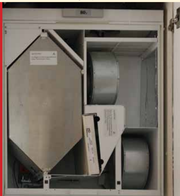
Ventilation unit with heat exchanger exposed
