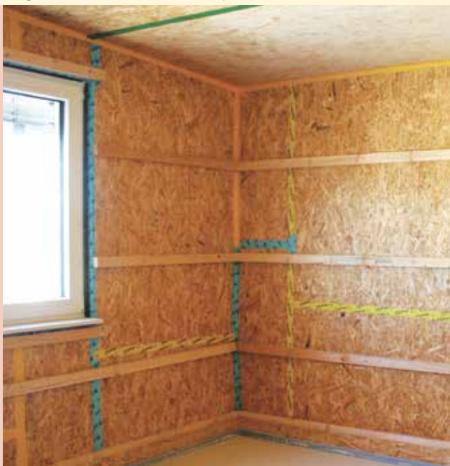
Airtight connections between wood composite boards
