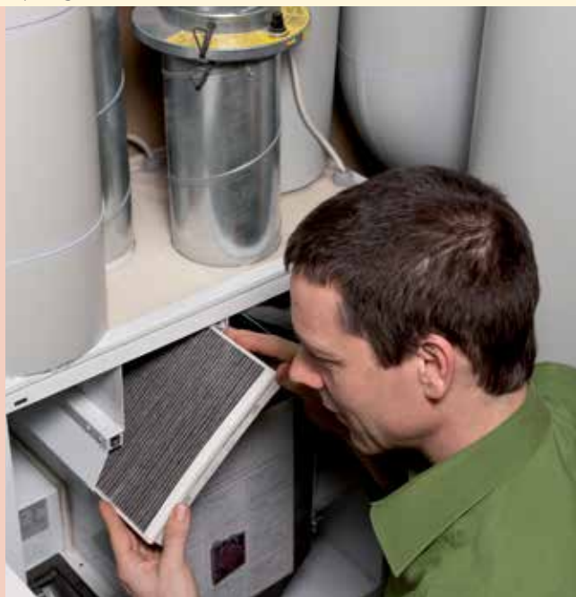
Replacing the filter of a ventilation unit.
