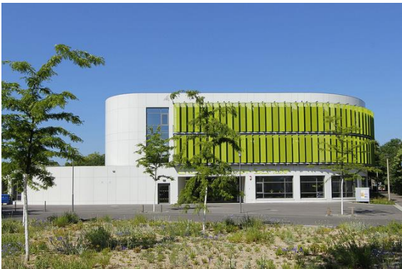
School in Leipzig built to the Passive House Standard, which was visited by conference participants within the framework of an excursion. Picture: City of Leipzig
