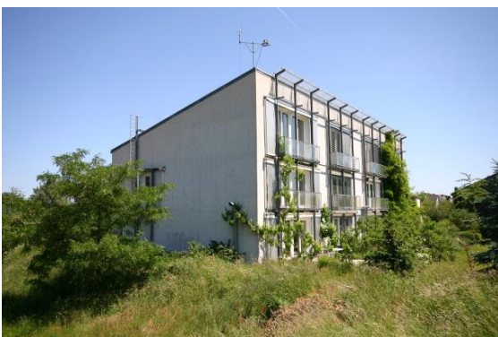
The world's first Passive House can be visited within the framework of the Conference. Photo: Passive House Institute
