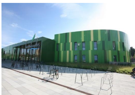
New Passive House leisure pool in the German city of Bamberg. Photo: Passive House Institute
