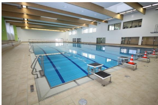
A particularly pleasant quality of indoor air is ensured in the sports area due to the Passive House Standard.
