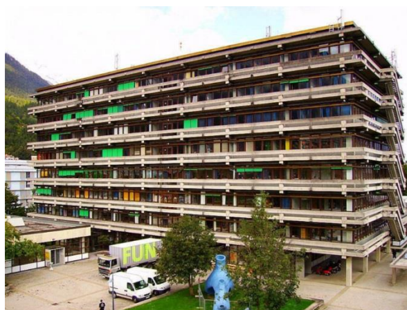
The university building in Innsbruck before the start of the refurbishment. Photos: Passive House Institute
