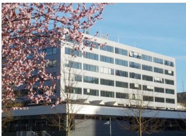
Energy efficiency and living comfort were improved significantly with an integrated planning approach.
