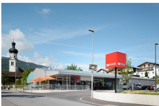
The new Supermarket in Passive House Standard in Natters near Innsbruck. Photo: MPREIS
