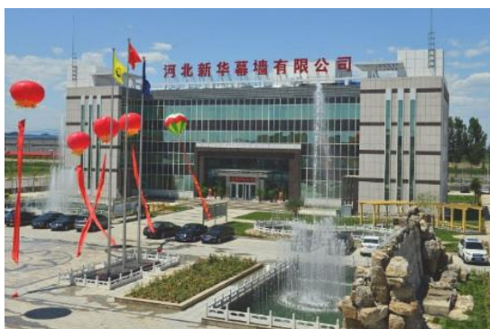
China's first office building in Passive House Standard. Picture: Schöberl & Pöll GmbH
