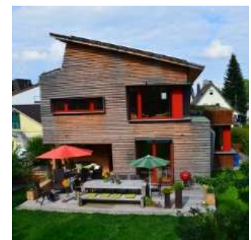
A Passive House in the Black Forest region in Germany.
