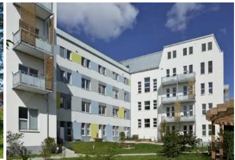
A residential building in Hamburg, certified to the EnerPHit Standard for refurbishments. Photo: Markus Tollhopf
