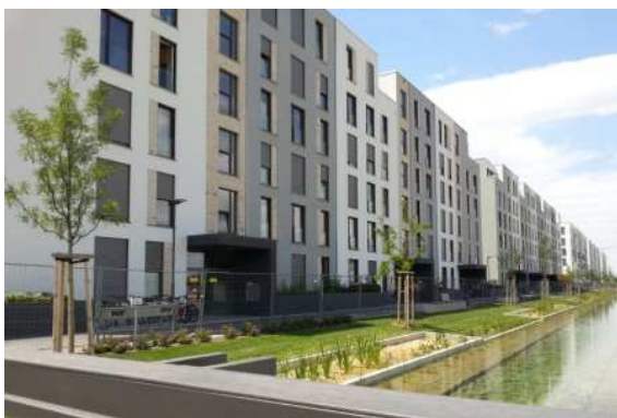
Hundreds already live in Bahnstadt, the new Heidelberg city district. Photo: Passive House Institute
