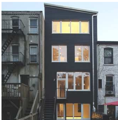
Tighthouse Retrofit (New York, USA). Photo: Hai Zhang
