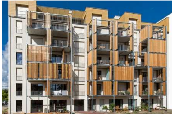
Boyen Street Zero-Emissions Apartments (Berlin, Germany). Photo: Deimel Oelschläger Architekten
