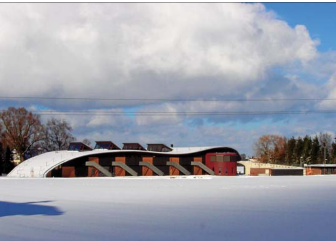
(opposite) This passive house montessori school, near Munich, breaks most of the preconceived expectations people have of this exacting standard; (top) the upper floor receives plenty of natural light through the expansive rooflights that punctuate the undulating green roof (above, right and below), which eventually rolls down to converge with the fields below
