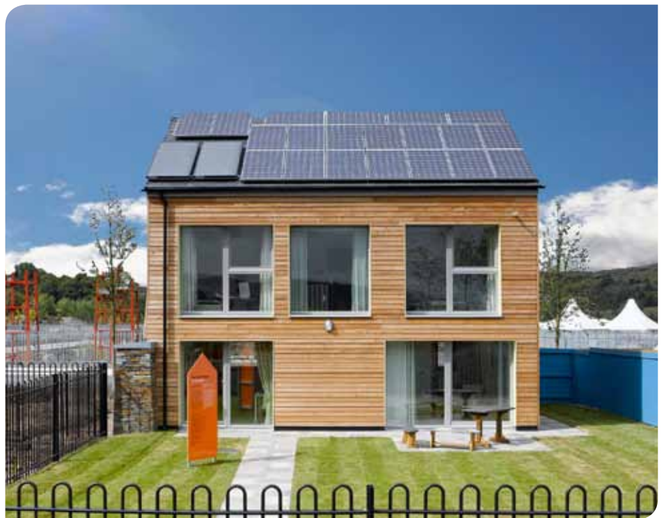
Figure 3 The Larch house, Ebbw Vale
