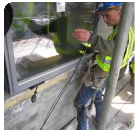
Figure 5 Window frame installation
