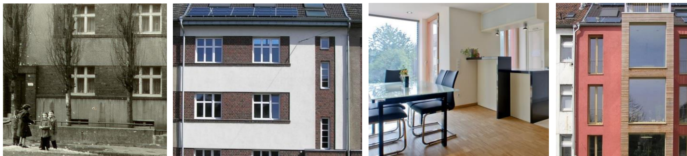
This 1930s building on a housing estate in Mönchengladbach, Germany, was retrofitted to the Passive House Standard. The garden façade has been transformed beyond recognition, Passive House database ID 5765. © bau grün! architekten
