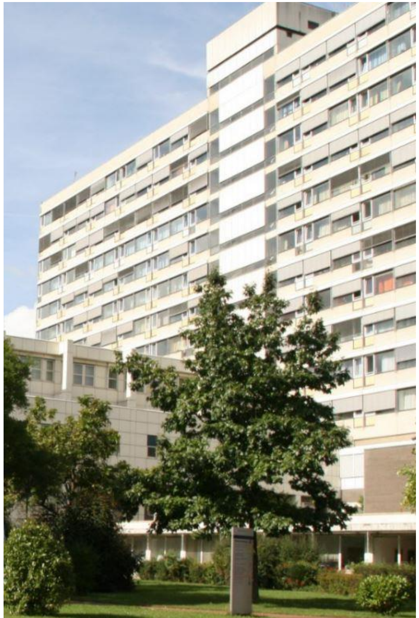
The existing building of the Klinikum Frankfurt Hoechst built in the 1960s. Among other things, the new Passive House Standard building will drastically reduce running costs. © Klinikum Frankfurt Hoechst
