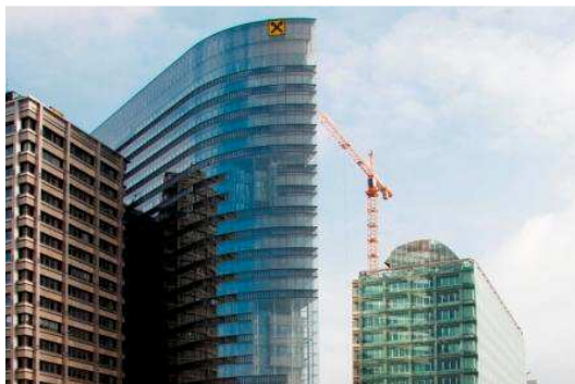
High-rise building with Passive House Certificate: the new office of the Raiffeisen-Holding NÖ-Wien. Image: IBO
