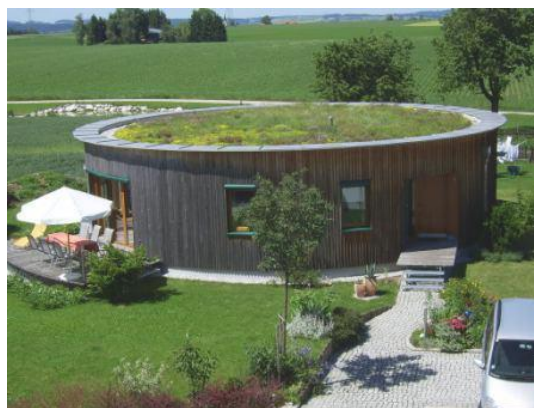
Passive House in Roitham, Austria that will be opening its doors to the public. Picture: Günter Lang
