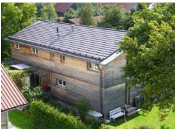
Also participating: a residential house in Biburg-Alling in Bavaria. Picture: Justus Well
