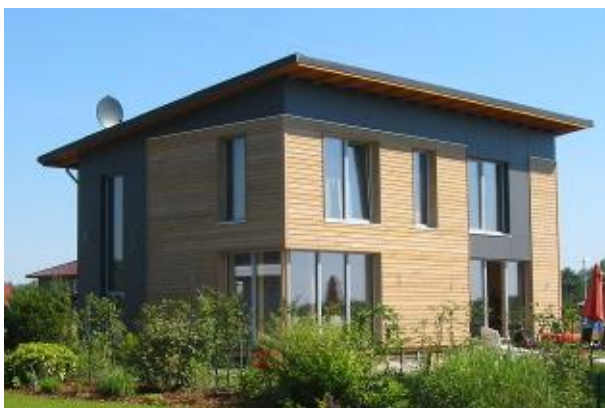
A Passive House in Westerstede in Germany which can be visited from 13-15 November. Picture: Christian Gauler
