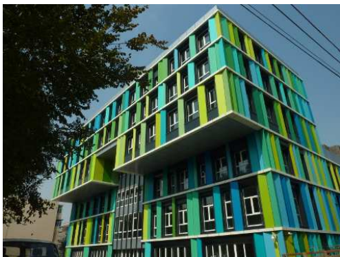
This new building in China will also be open to the public during the international Passive House Days. Photo: Passive House Institute
