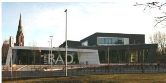
Full view of the Passive House swimming pool in Lünen near Dortmund, open since 2011. Photo: PHI
