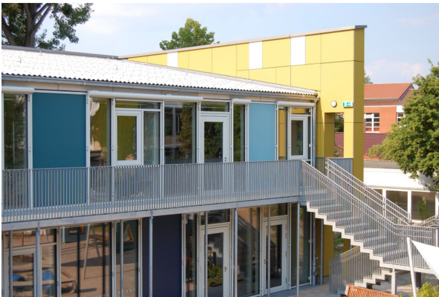
A Passive House kindergarten in Hanover-Linden, supported with 47,500 euros by eneracity-Fonds proKlima, Source: proKlima/Glombik.
