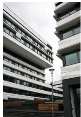
Office building in Heidelberg's new Bahndtadt quarter. Photo: PHI
